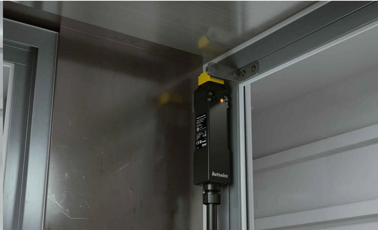
Door lock switches can be used to prevent door being opened during equipment operation.
