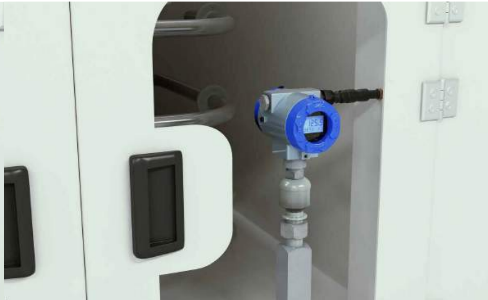
Pressure transmitter are used to check the hydraulic pressure of the solution in the pipe and transmit the current value.
